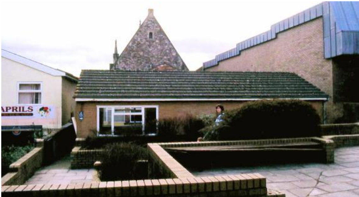
The old 2 roomed extension about to be demolished
